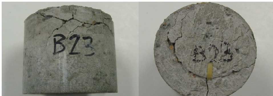
Figure 3-17 Cracks due to Differential Thermal Expansion
