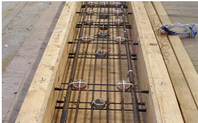
Figure 5-9 Layout of Sensors and Steel Reinforcement
