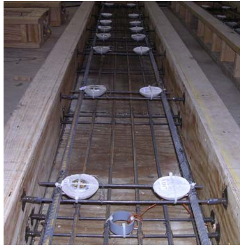
Figure 7-10 Layout of Sensors and Steel Reinforcement
