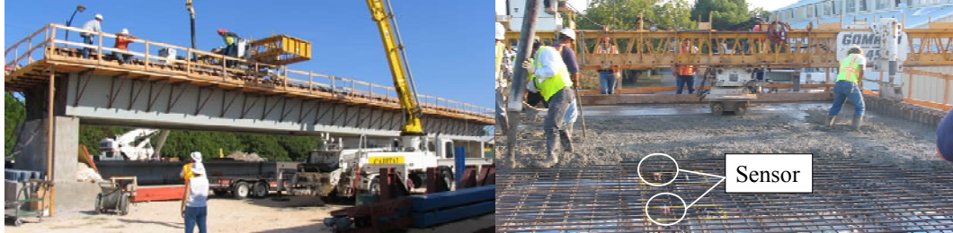
Figure 8-7 Sensors Embedded in Full-Scale Bridge Deck
