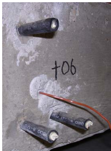
Figure 5-7 Sealed End of Transverse Reinforcement
