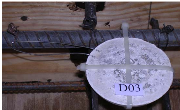
Figure 7-12 Sensing Wire Placed out of the Expected Path of the Crack
